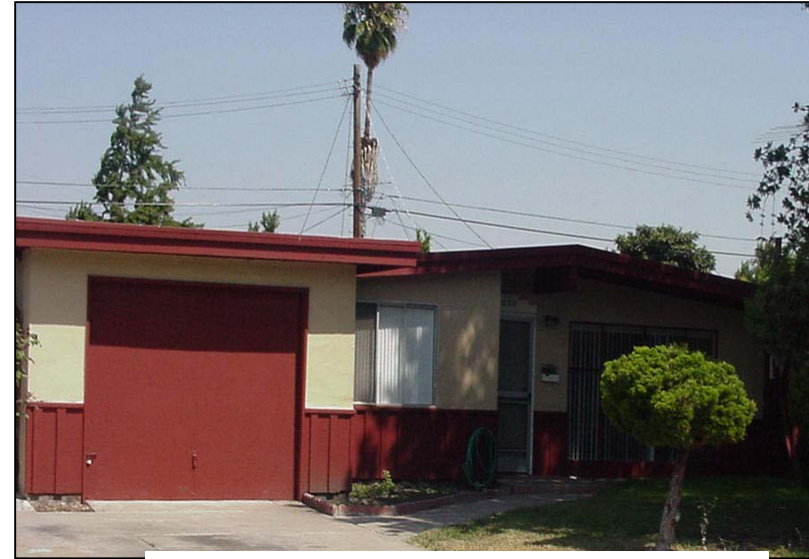
A Typical Mid-Century style – Not of the area.
